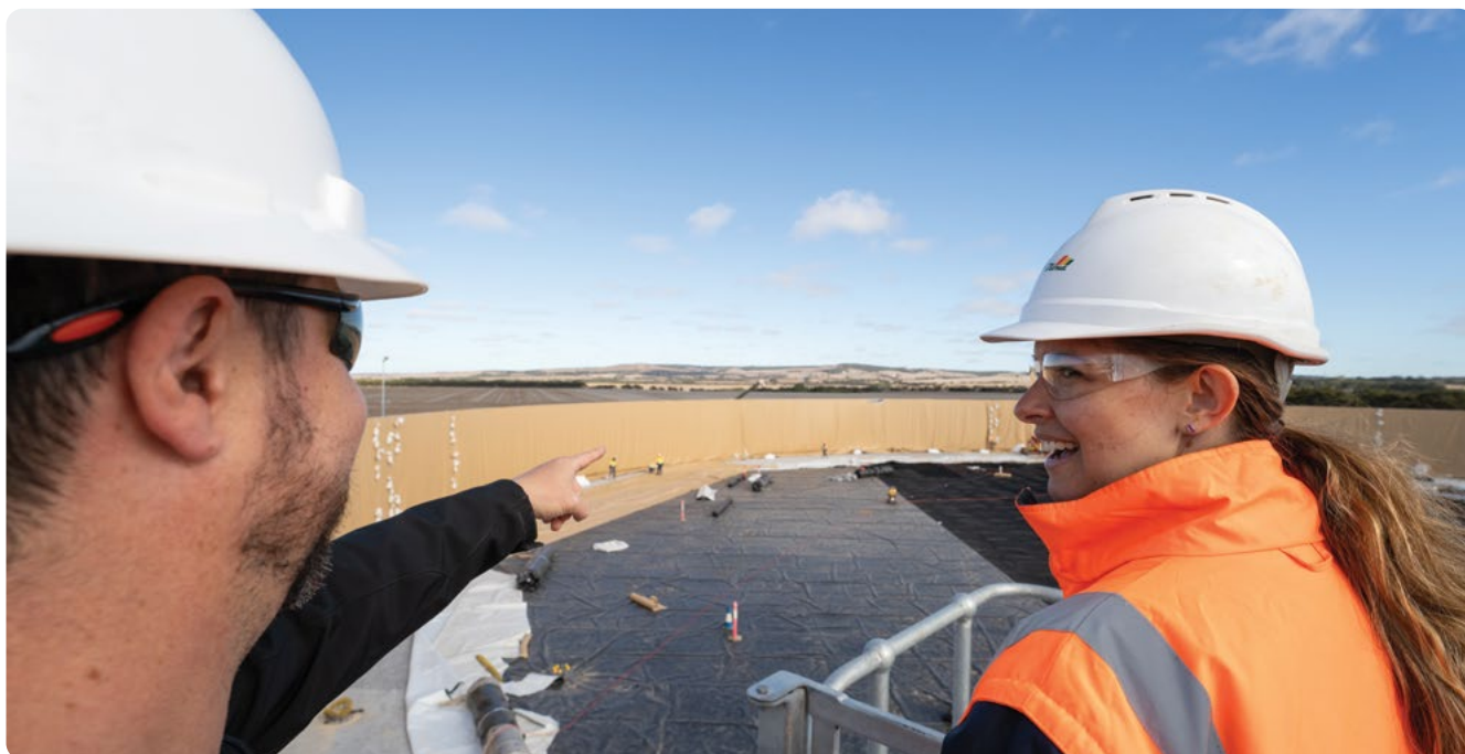
Overlooking the construction of water tanks at the Summit.
