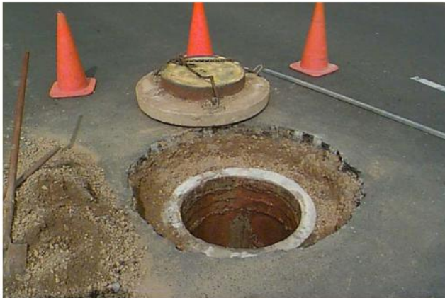
Figure 3. Typical Excavation (for casting adjustment)
