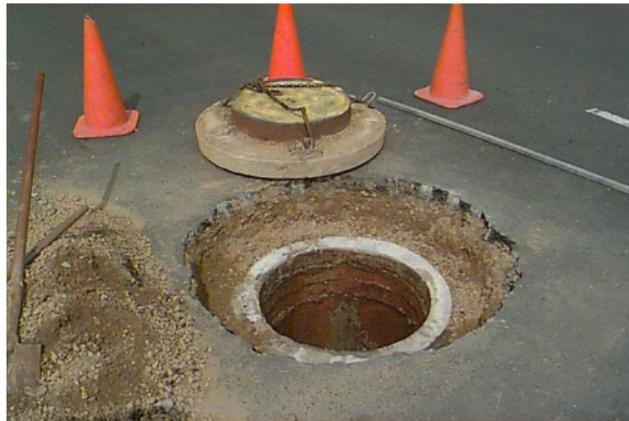
**Figure 3. Typical Excavation (for casting adjustment)**
