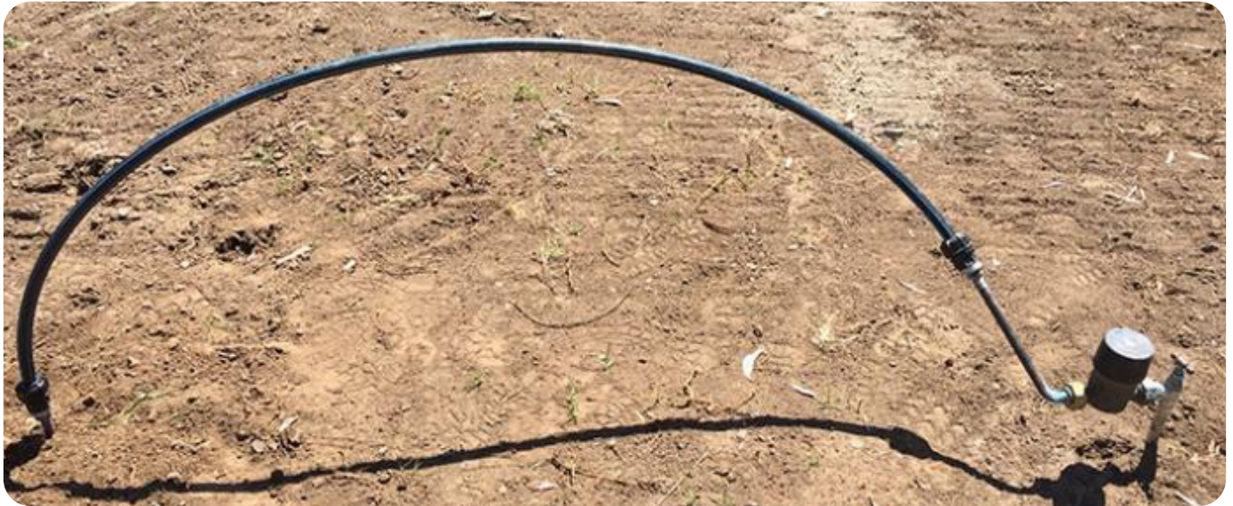
Example of temporary connection to your plumbing
