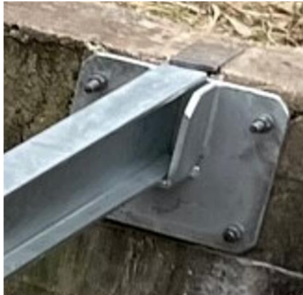
Figure 3: Steel beam – wall connection
