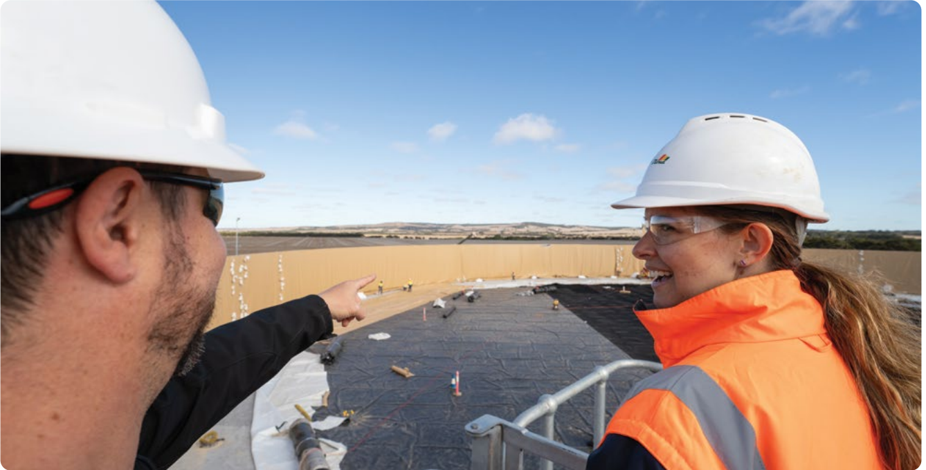
Overlooking the construction of water tanks at the Summit.
