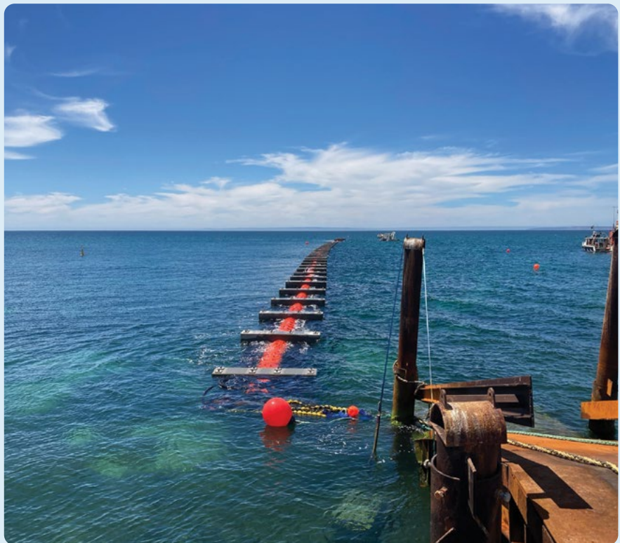
A section of pipeline being laid off the coast of Penneshaw.
