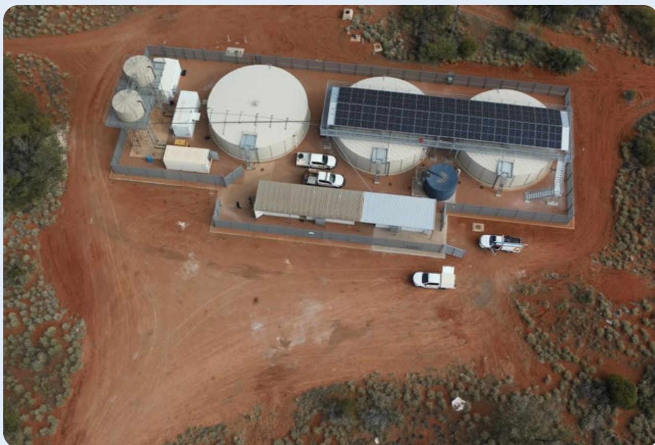
Kaltjiti Desalination Plant with solar panels.
