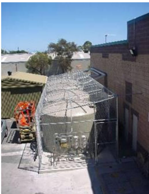
Aerial view of the storage tanks
